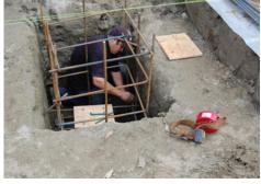
Carpenter tying the steel footing dowels for the steel columns canopy.
