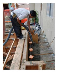
Pouring the elevator pit walls and footings
